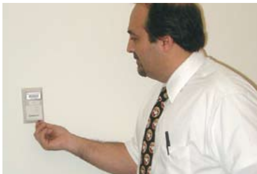
The Smart Sensor provides facilities staff a convenient way to adjust room temperatures
