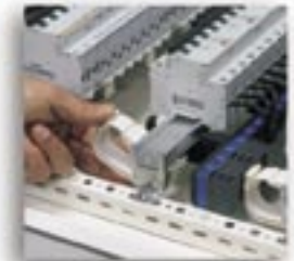
Wiring straps are clipped onto the back of the modular rail.
