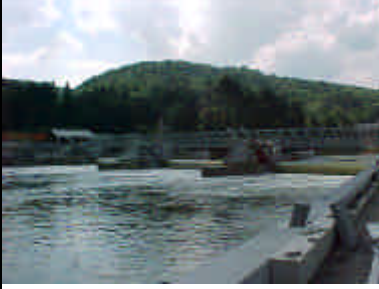
New dam in Anseremme
